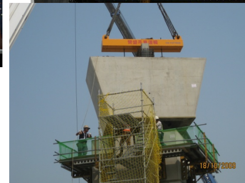
Installation of column cap
